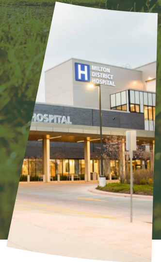
Milton District Hospital 8-minutes by car
